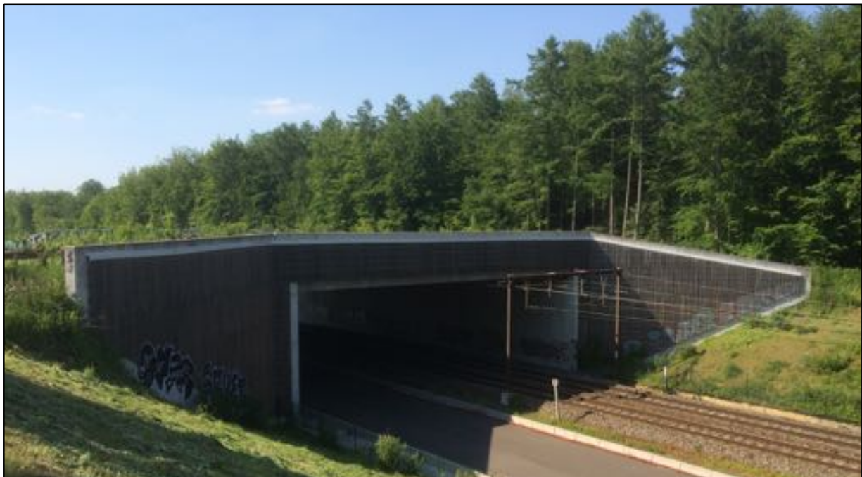
Image 5: Green Bridge across a new high speed rail line near Brussels; this was constructed to allow movement of mammals and ecological connectivity across the railway between two nature hubs (woodland blocks) hence avoiding animal collisions, damage to rolling stock and line disruption. Such an approach should be advanced for HS2.
